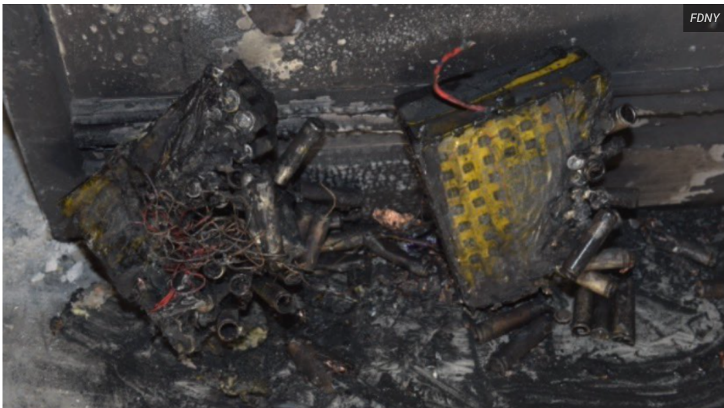
Charred remains of an electric bike batter shared by the New York City fire department.
